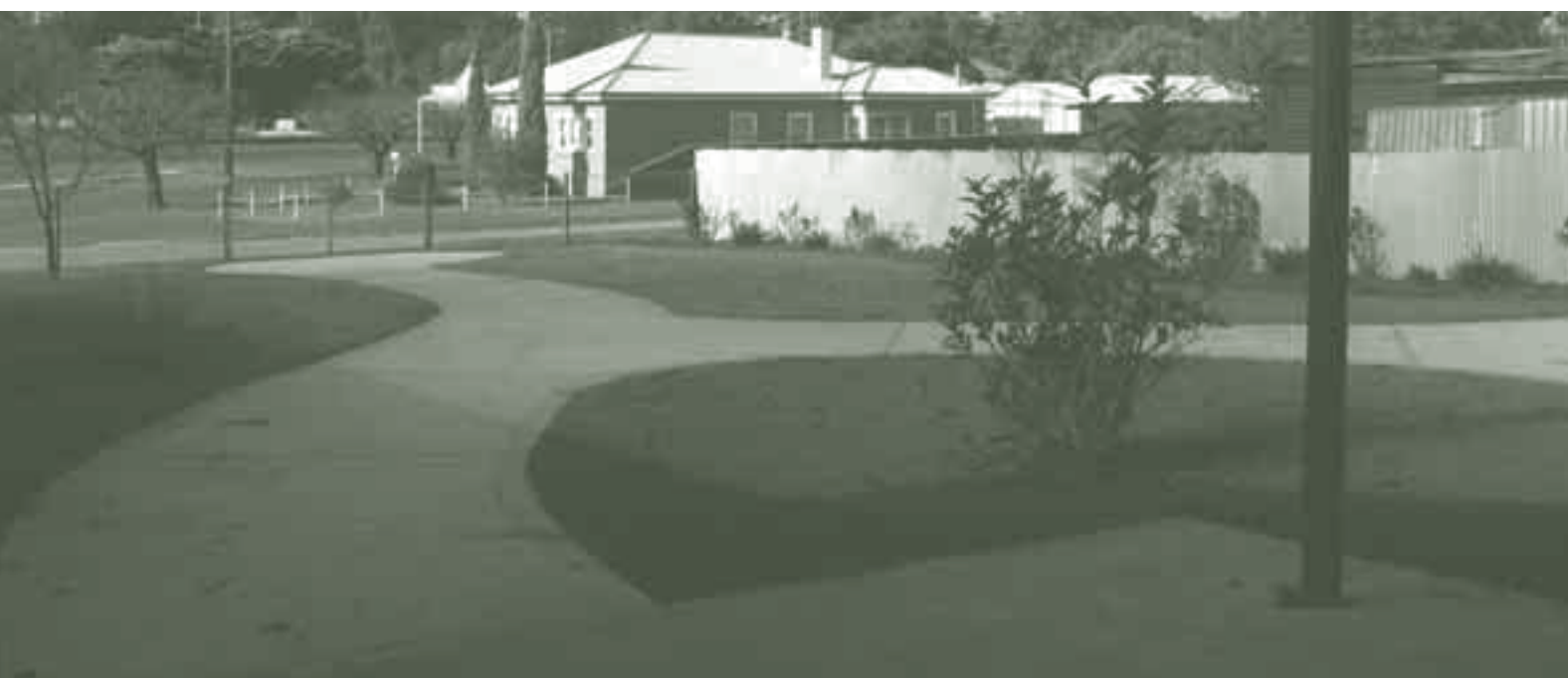
New paving for the Beaufort Hostel
